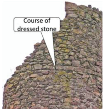
Extended tower and stone course
