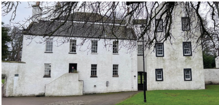
The Walltower House; the old croft has become a three-storey addition on the right
